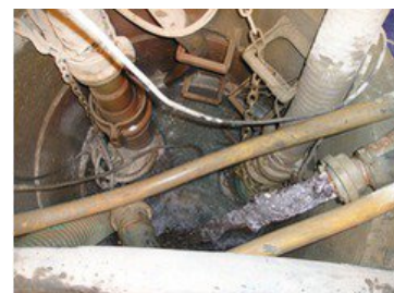
Collecting shaft with KTZ47.5 and KTZ35.5 in operation in snore mode
