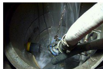
Collecting shaft with KTZ47.5 and KTZ35.5 in operation in snore mode
