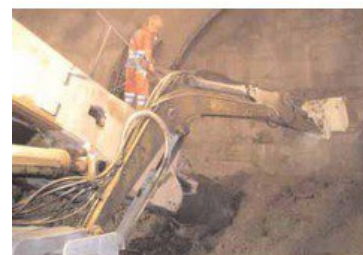
Portal with partial cut machine in operation
