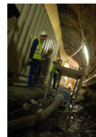
Dewatering using a Tsurumi-Boosterpump
