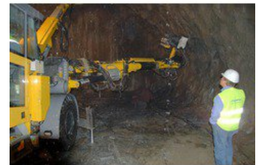
Water amount in the tunnel clearly visible, KRS in the background
