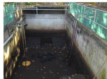
Iseltwald wastewater plant, Switzerland - FHP pump in aerobic treatment tank
