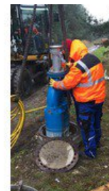
Plenty of space in the shaft for the dry run-protected KRSU that runs on 3-phases with 400V via a direct start and fits into most German access shafts (Photo: Tsurumi)
