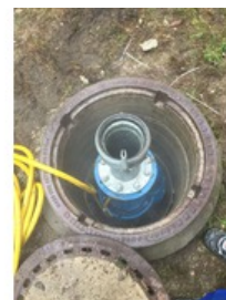
Looking at the centred DN200 pressure nozzle (Photo: Tsurumi)
