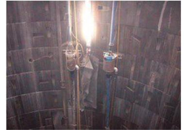
Vertical Pumps: "Riser pipes in the supply shaft: Four small Tsurumi pumps installed in series are all that's needed to ensure drainage vertically upwards through the tunnel"
