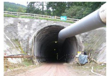
900 metre stretch of pumping in "The Bleßberg Tunnel: chains of pumps reaching 900 metres and more are possible when connecting pumps in series"
