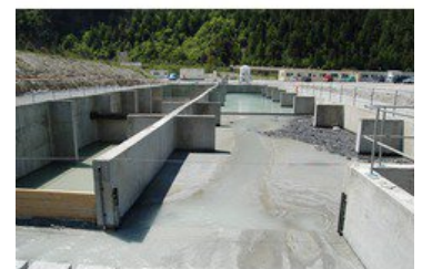
Mud from the tunnel water in the sedimentation basin
