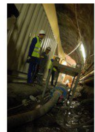
Dewatering using a Tsurumi-Boosterpump
