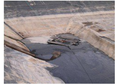
Pumps submerged in leachate basin
