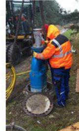
Plenty of space in the shaft for the dry run-protected KRSU that runs on 3-phases with 400V via a direct start and fits into most German access shafts (Photo: Tsurumi)
