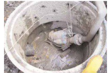
Shaft ring dewatering
