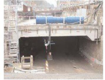
Tunnel entrance Hermann-Lönsstraße, 1st section of excavation.
