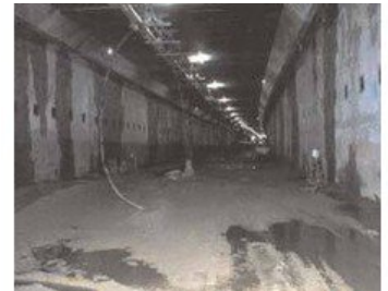
View into the tunnel, 3rd section of excavation.
