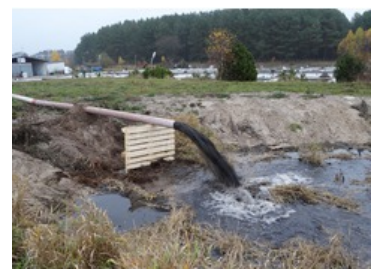
The sludgy mixture is channelled through a hose to the sedimentation tank (photo: Tsurumi) Download photo
