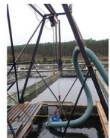
The submersible pump hangs on a chain, meaning it can be freely positioned (photo: Tsurumi) Download photo
