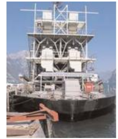
Front view of the two screening plants
