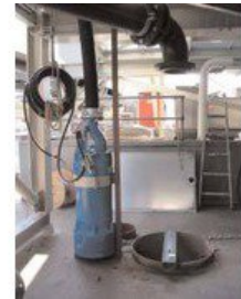
LH430 prior to installation in shaft
