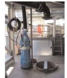
LH430 prior to installation in shaft
