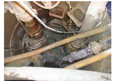
Collecting shaft with KTZ47.5 and KTZ35.5 in operation in snore mode
