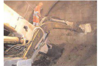
Portal with partial cut machine in operation
