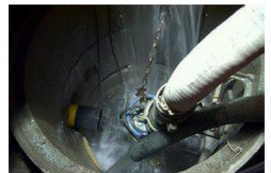
Collecting shaft with KTZ47.5 and KTZ35.5 in operation in snore mode
